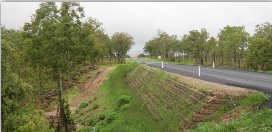
Photo: Completed GCS Wall with the first signs of vegetation
