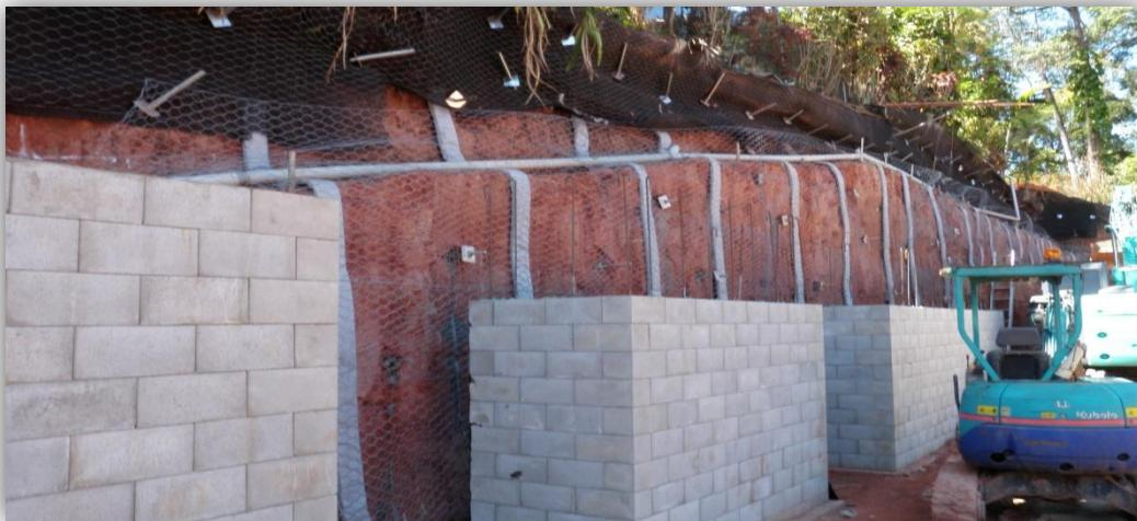
Photo: Complete composite GCS & block retaining wall system ready for landscaping.
